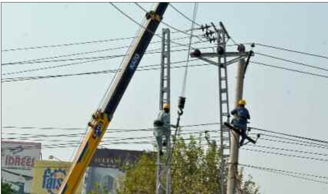
LAHORE: LESCO staffers install new electric wires at a pole.
