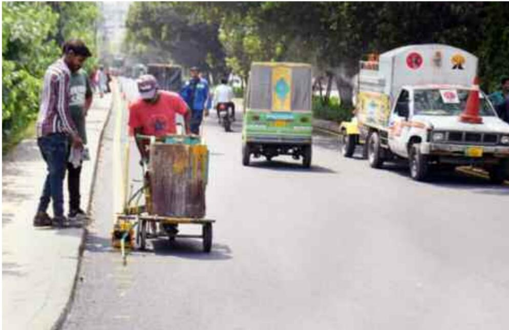
LAHORE: Worker lays down yellow boundary lines with the help of a machine on Model Town Street. —Online
