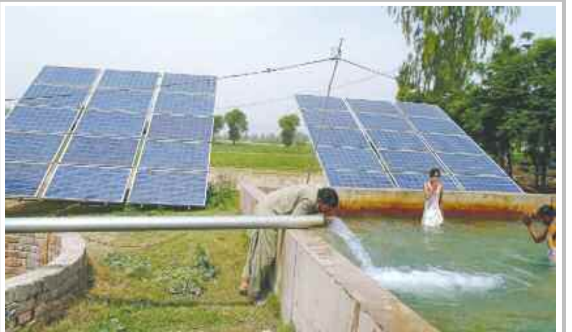
CHINIOT: A man drinks water from solar panel system tube well. Demands of solar system increases in country in Agricultural Sector.
