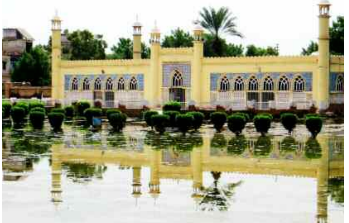
HYDERABAD: A view of reflection of Main Eid Gah in accumulated rain water as drainage has not been started and attention for concern authority. —Online
