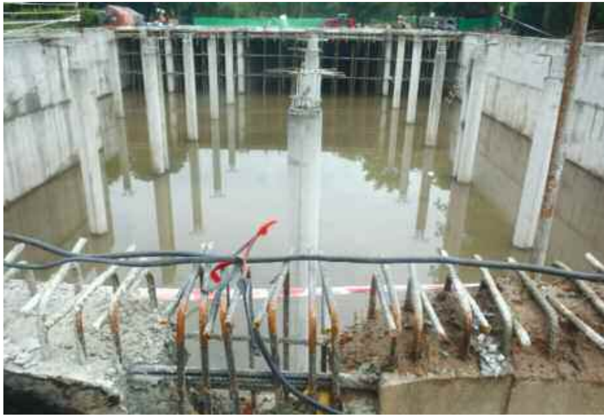
LAHORE: A view of under construction paved ditch for accumulating 15 thousands cans water on Larnce Road as constructed by WASA for agriculture purpose. —Online
