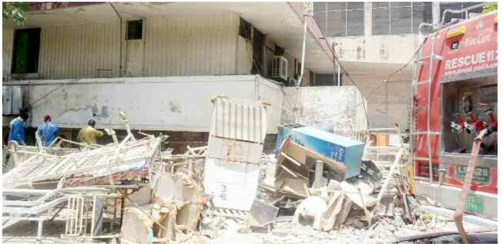
LAHORE: A view of debris as after fire erupted due to short-circuit in the surgical emergency ward of Services Hospital as around 40 patients are being treated there and all of them have been rescued. —Online
